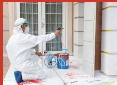
NP refresh service exterior wall paint spraying
