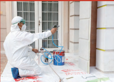
NP refresh service exterior wall paint spraying
