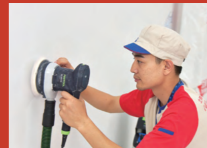
NP refresh service wall polishing
