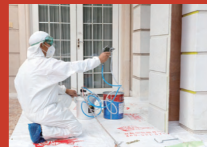
NP refresh service exterior wall paint spraying
