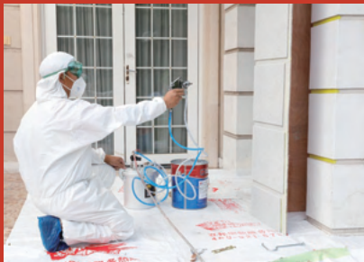
NP refresh service exterior wall paint spraying
